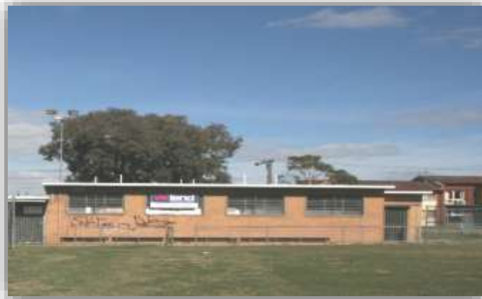
Hadfield F.C. Change rooms | Built 1960's | Reddish Reserve
